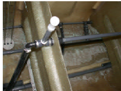
Fig.3: inside of tank is cleaned by two rotating nozzles on the splash walls (baffles).
